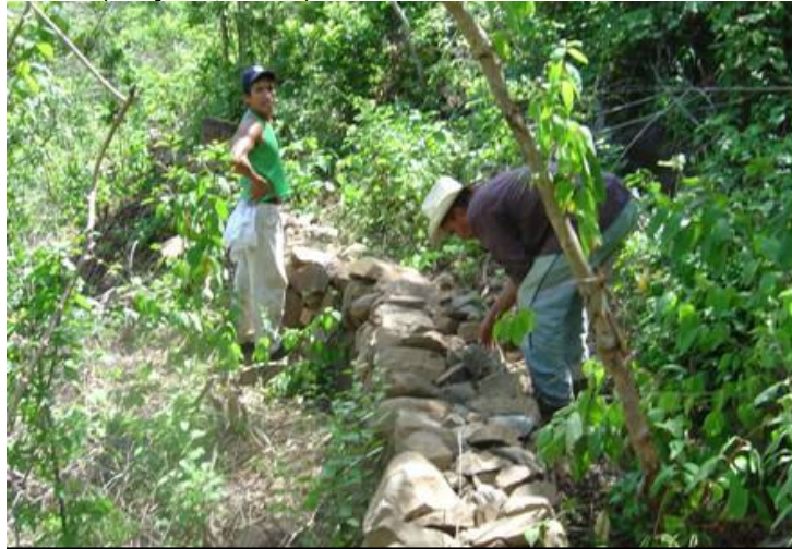
Figure 4. Farmers under PES contract building rows of stone barriers to enhance water infiltration and decrease soil erosion (May 12, 2005)
