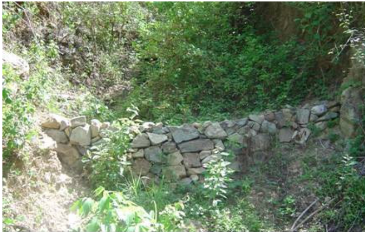
Figure 3. Stone ditch enhancing water infiltration and avoiding soil erosion in a creek located in the water catchment area in Paso de Los Caballos micro watershed, San Pedro del Norte (May 12, 2005)
